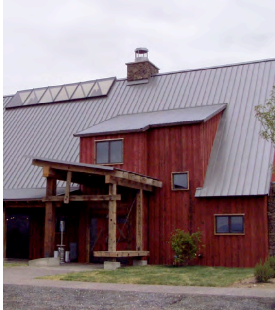
Figure 1 – Unpainted Bonderized steel roof (courtesy of Steelscape Inc.)
