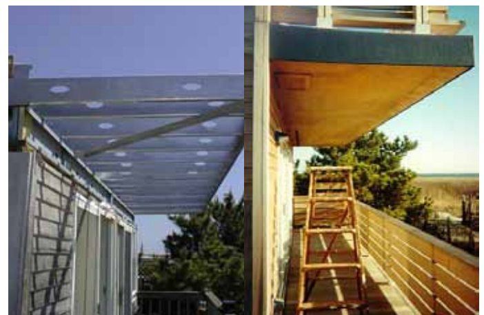
Figure 9 - New Jersey Site Under Construction
