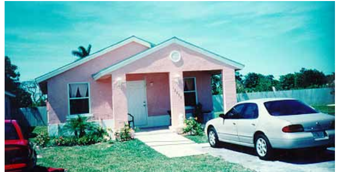
Figure 2 - Miami, Florida Corrosion Site
