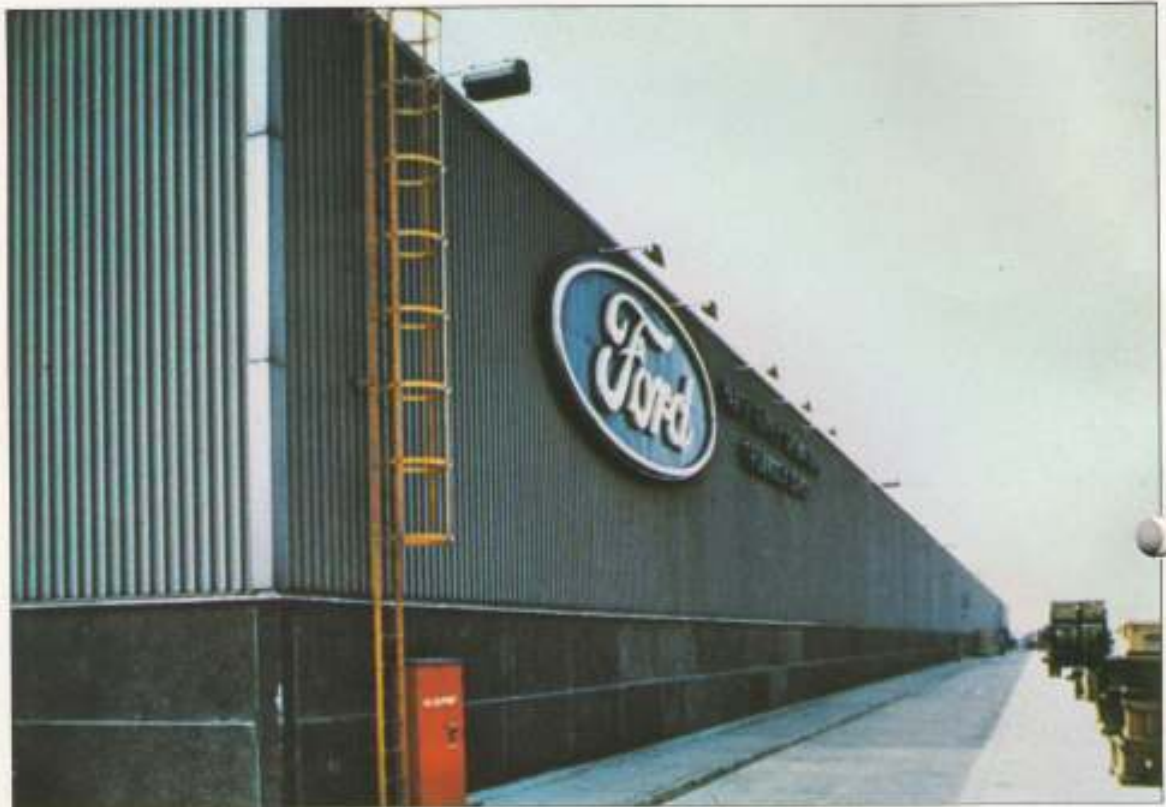
Fig. 7 Ford Motor Company Parts Depot at West Thurrock, Essex.
