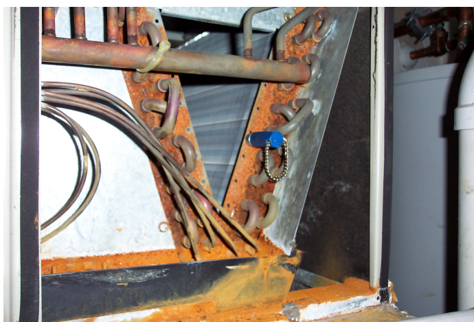
• Photo 1 Galvanic (bimetallic) corrosion in A/C unit
