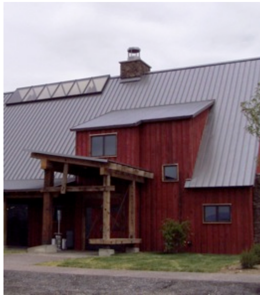
Figure 1 – Unpainted Bonderized steel roof (courtesy of Steelscape Inc.)
