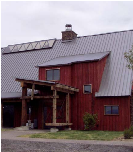
Figure 11 – Unpainted Bonderized steel roof (courtesy of Steelscape Inc.)
