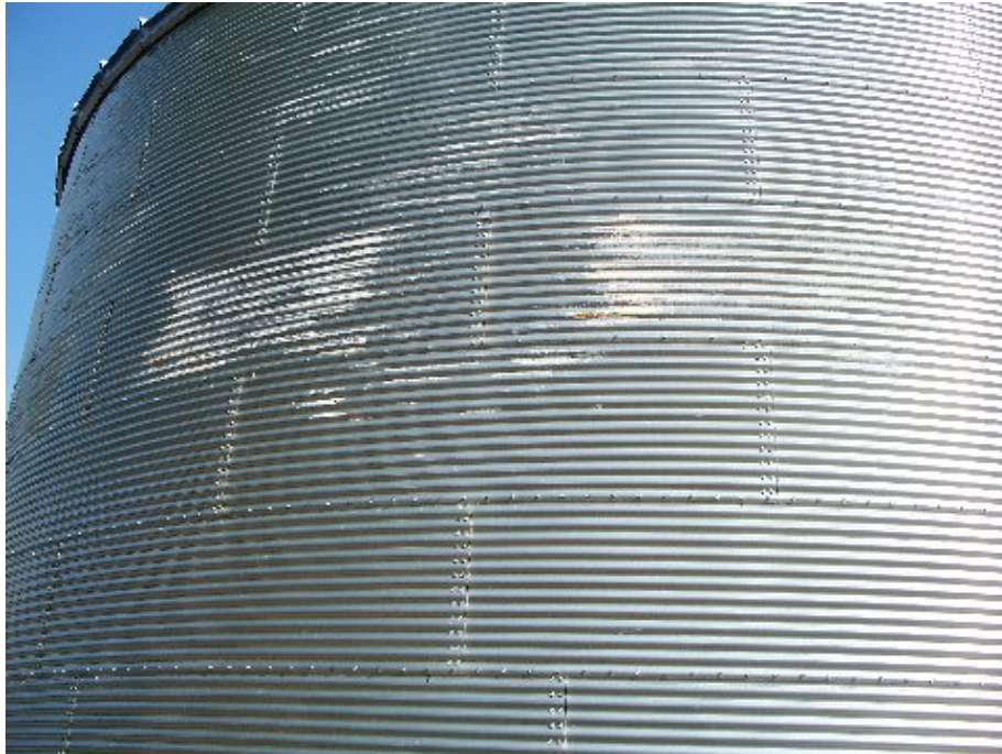
Storage stain on grain bin panels 3 years after erection (July 2010)
