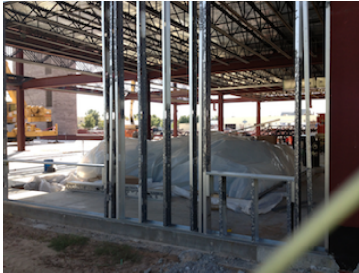
Black storage stain on installed framing (September 2013)
