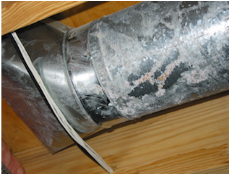
Corroded residential ductwork (March 2005)
