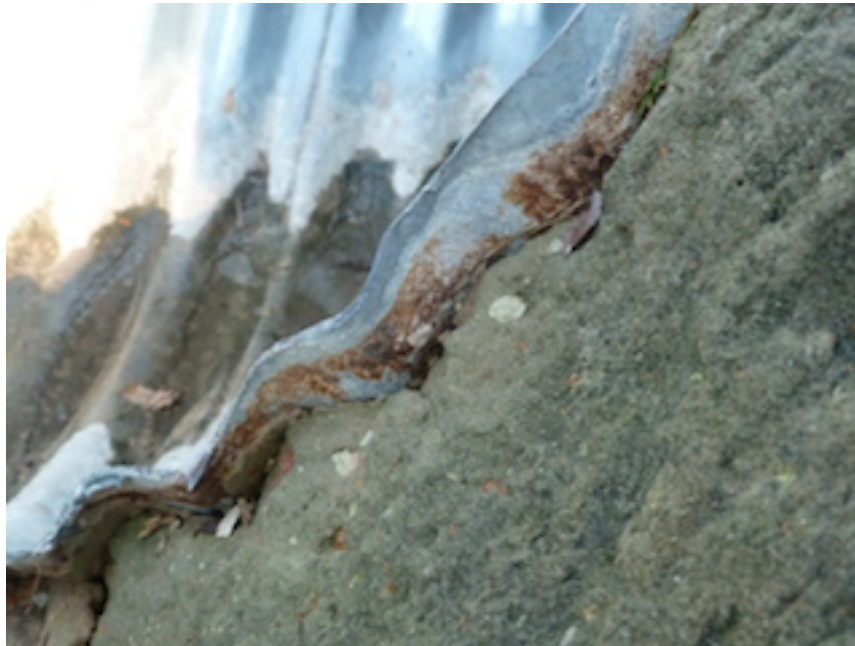
Soil-side corrosion on culvert pipe (January 2012)
