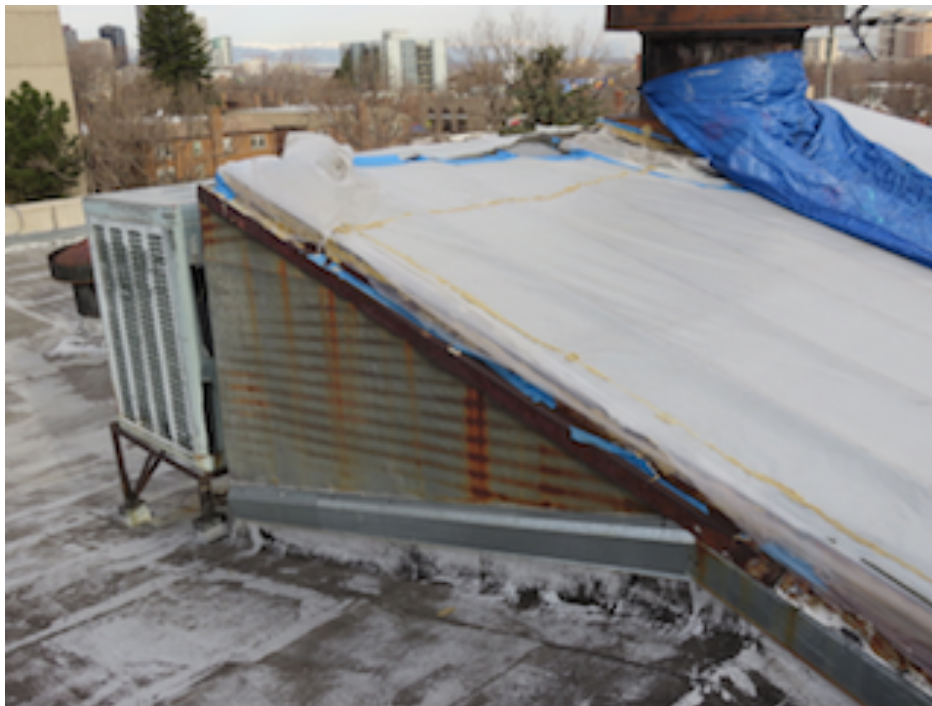
Corroded galvanized roof structure in Denver (August 2017)
