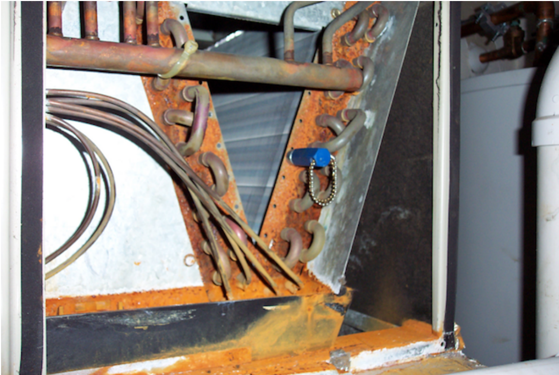
Galvanic corrosion of A/C unit galvanized end-plates and frame (October 2004)
