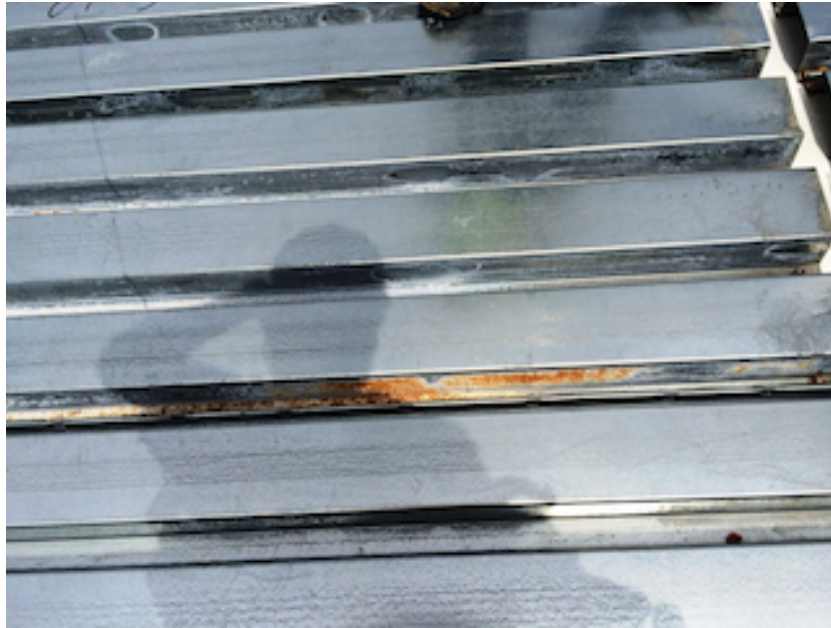
White and red rust on roof decking (October 2015)
