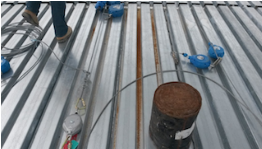
Red rust on the bottom channels of roof decking
