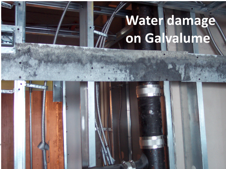
Water damage on galvanneal
