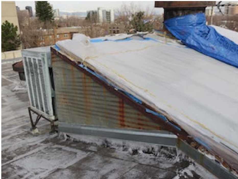
Corroded galvanized roof structure in Denver (August 2017)
