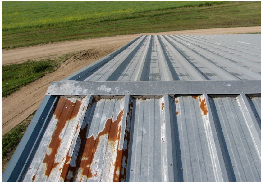
Corrosion on Farm Building Roof (August 2010)
