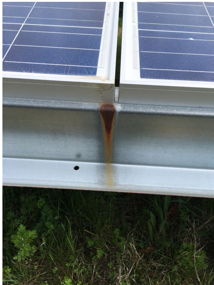
Corrosion of galvanized support of aluminium-framed solar panels (July 2018)
