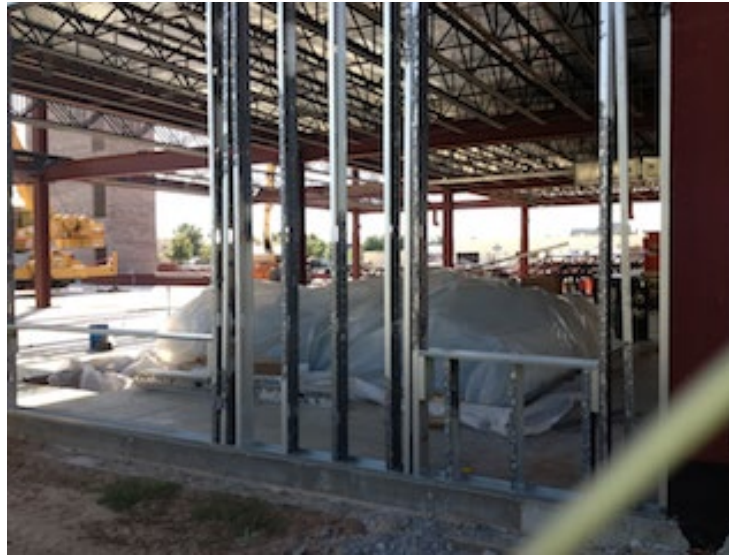
Black storage stain on installed framing (September 2013)
