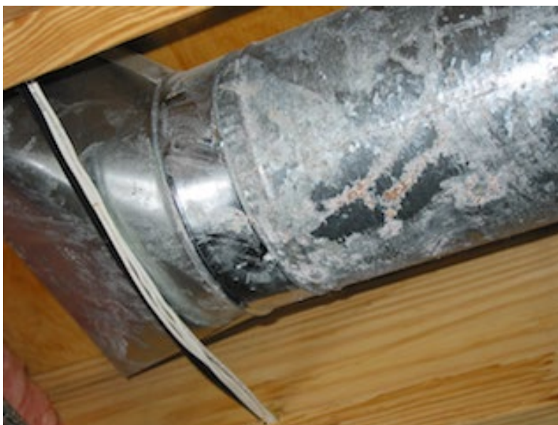
Corroded residential ductwork (March 2005)
