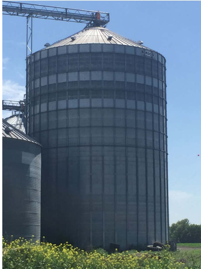
Uneven darkening of galvanized sheet panels on a large grain bin made with material from different lots (2019)
