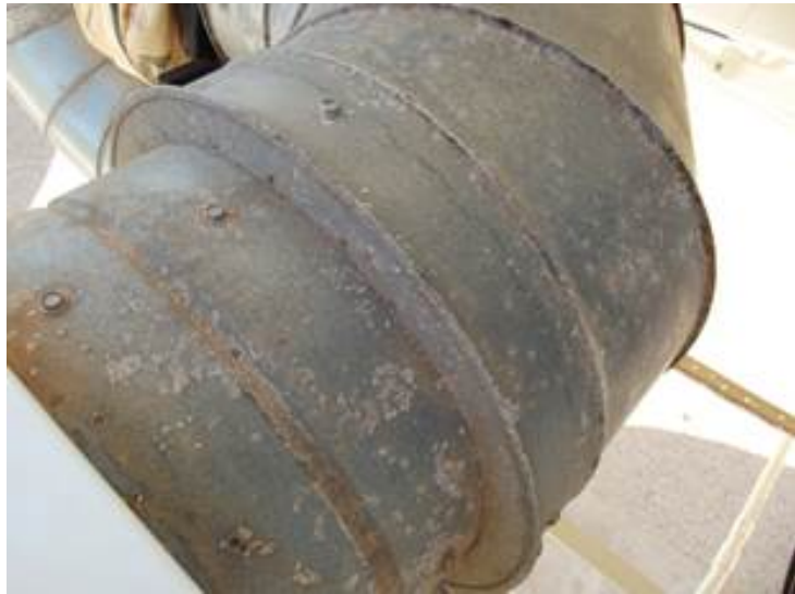
Surface of G90 HVAC located about 1 mile from the coast of Western Australia (October 2015)
