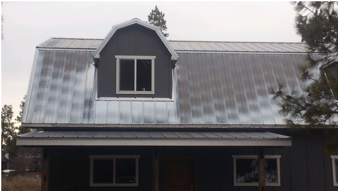
Uneven white rust formation on a G90 roof, 5.5 years old – west-facing exposure, Spokane, WA area (2019)
