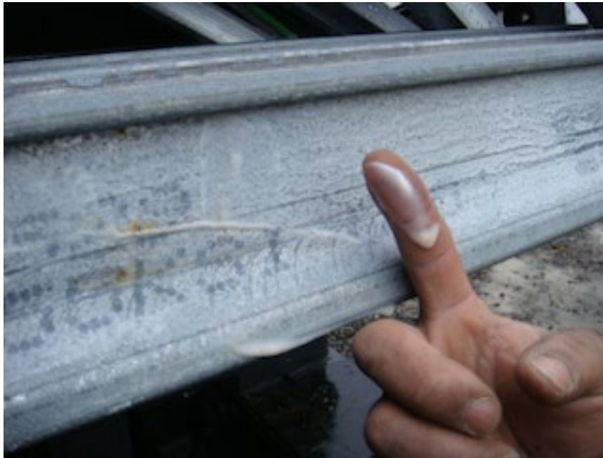
Unknown “foam” on framing after getting wet in the field (January 2008)
