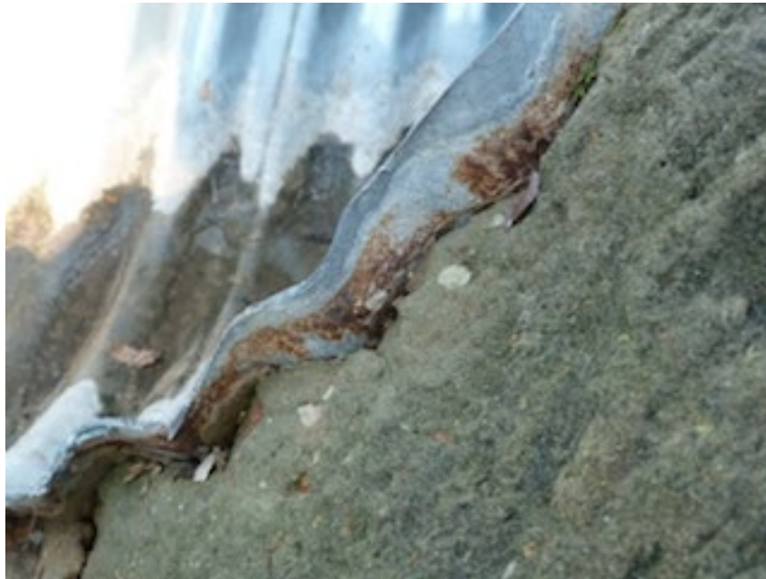
Soil-side corrosion on culvert pipe (January 2012)
