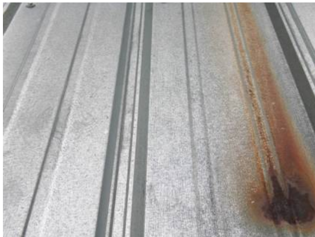
Rusted area from water draining off a wood fascia (May 2010)
