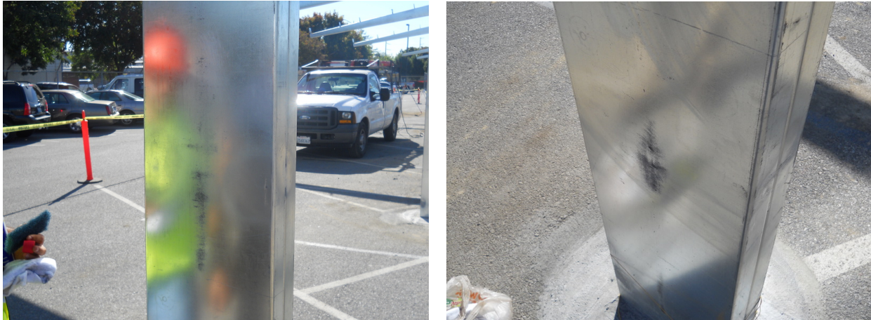
Fretting on Galvanized Poles (February 2012)
